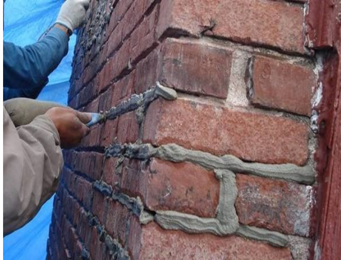
Fig1.11: Pointing wall
