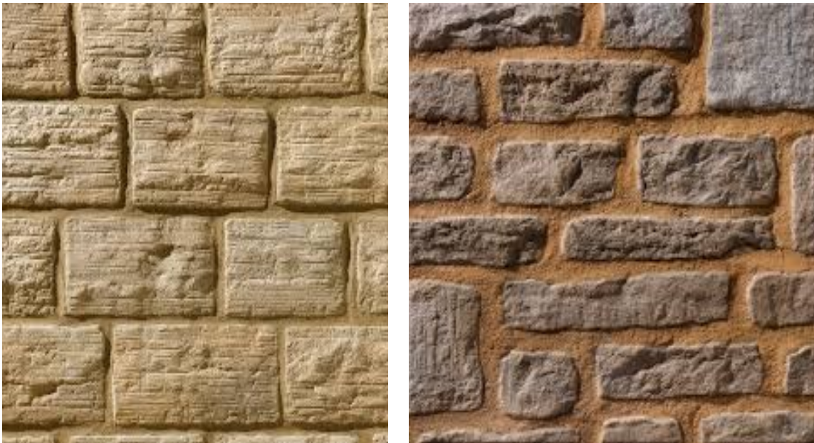
Fig.1.9 Random rubble masonry finished wall
