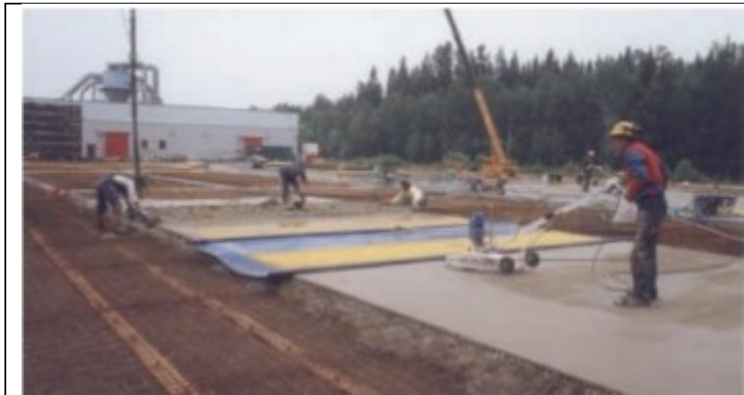
Fig.2.13: While vacuum is on, surface that has already been vacuum dewatered is floated with a power trowel fitted with a disc
