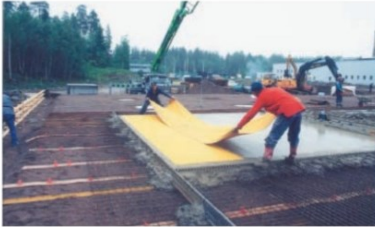
Fig:7-The filter pads are placed so that there will be a sealing edge around the entire filter pad surface
