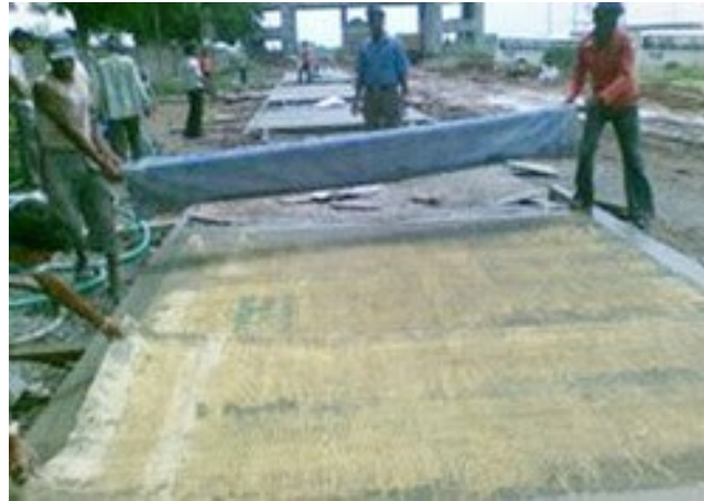
Fig 2.7 : Termix laying
