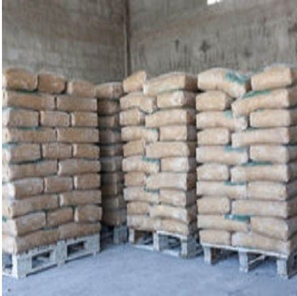
Fig 4.4 : Stacking of cement in Godown Fig.4.5:Stacking of bricks
